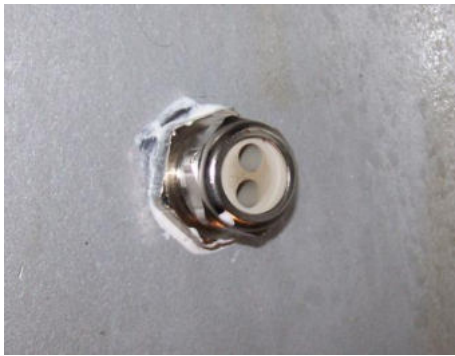
Fig. 24: Cable gland type B
