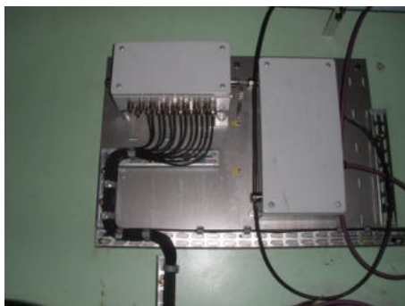
Fig.58: Mounting bracket BLG00402 with terminal box GHG002621... and one line converter box GHG002611...
